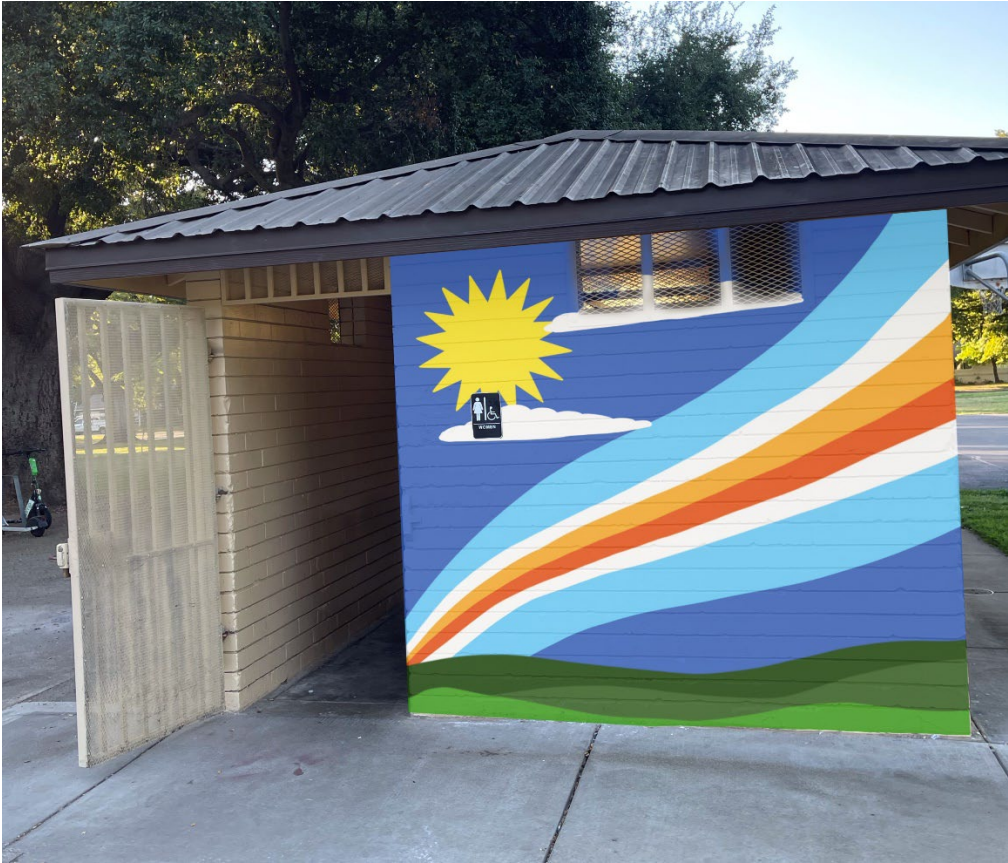
North Facing Wall
