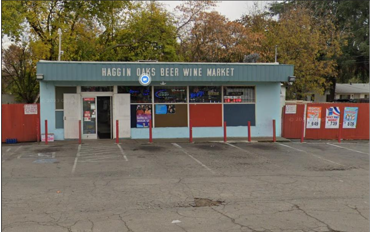
Figure 2: Existing Site Condition – Del Paso Boulevard Street Frontage
