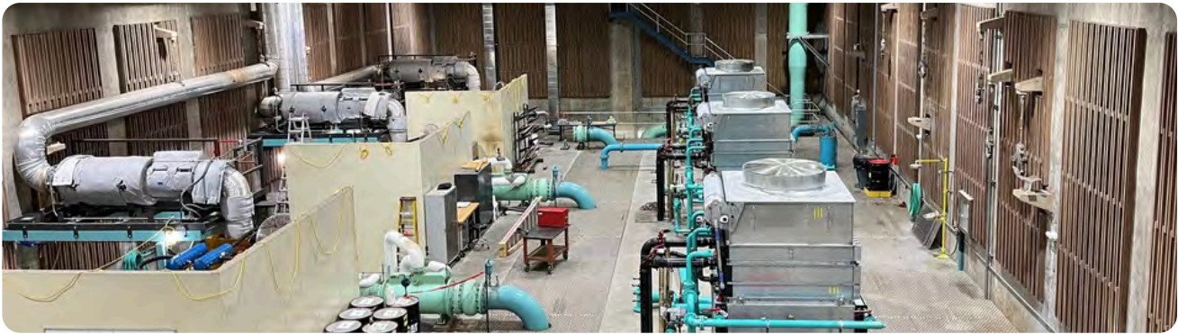
Florin Reservoir after LED lighting retrofit
