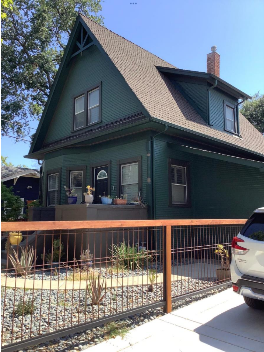
Photo 2: West facing street façade and south side of house with tool shed addition from 1964. The front door shown has been replaced with the original 1901 door.
