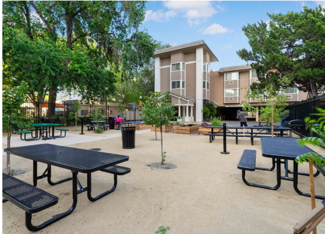
Central Sacramento Studios Phase 1
