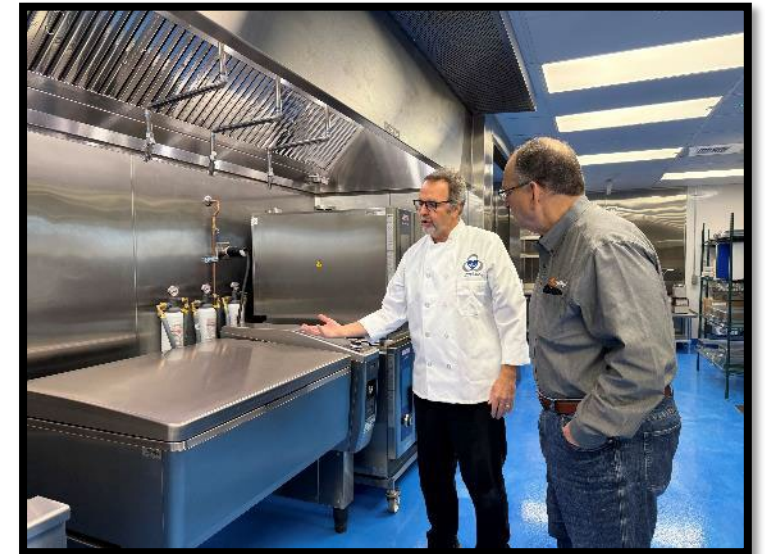
Existing Building Electrification
