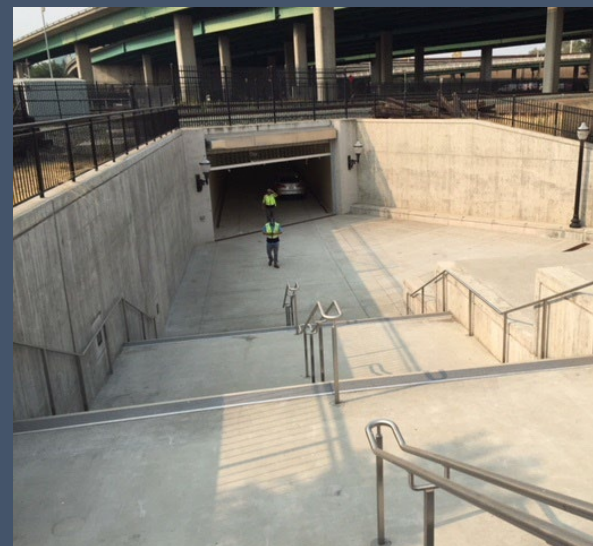
North of Tracks Stair and Ramp
