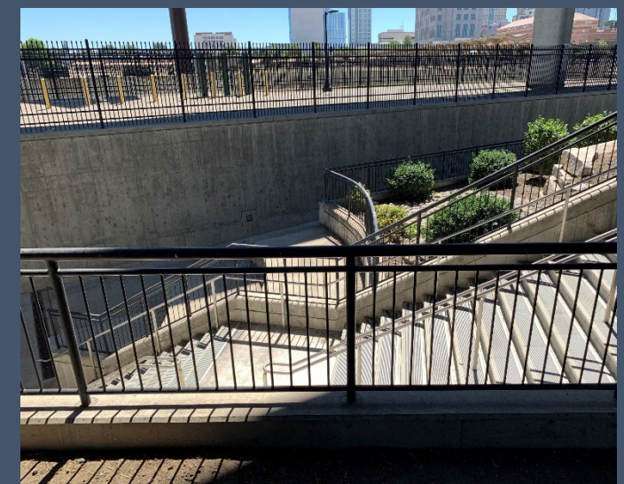
South of Tracks Stairs and Vehicle Ramp
