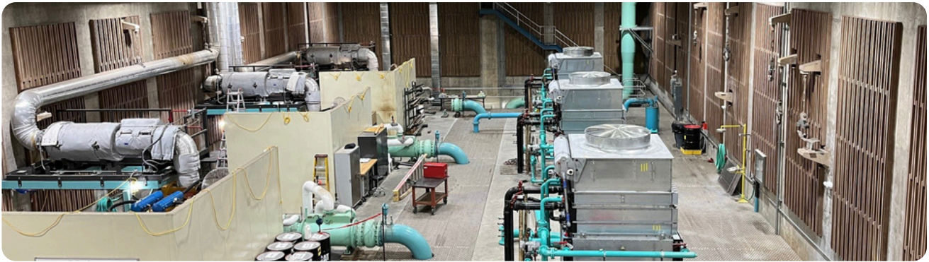
Florin Reservoir after LED lighting retrofit
