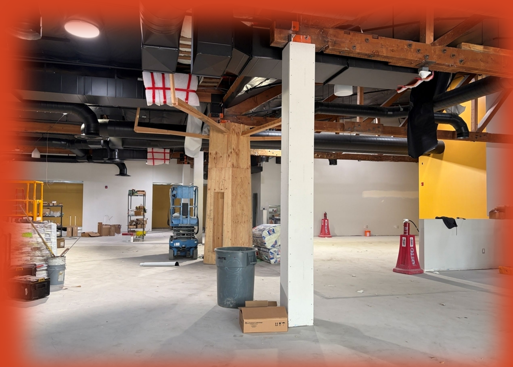
North Sacramento-Hagginwood Library retrofit
