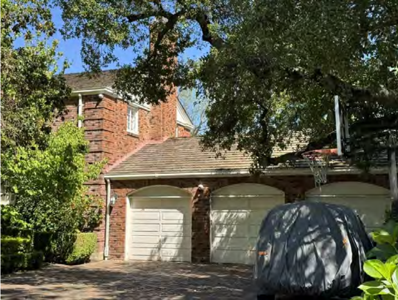
Photograph 3. View facing east, April 23, 2026.
