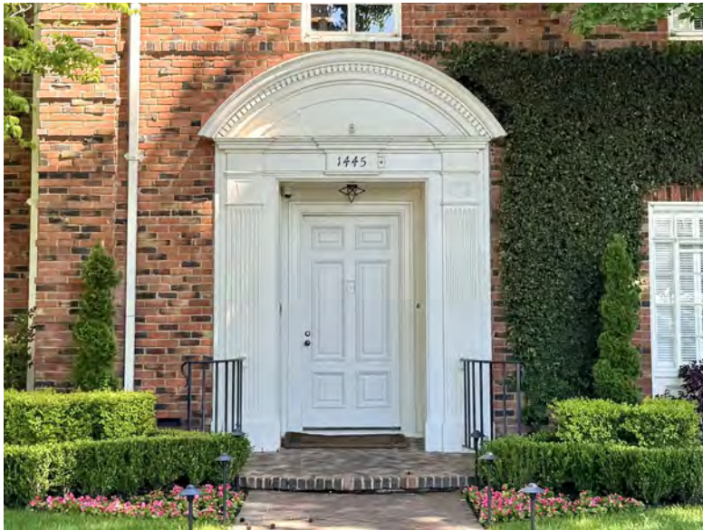
Photograph 1: View facing east, April 23, 2026.
