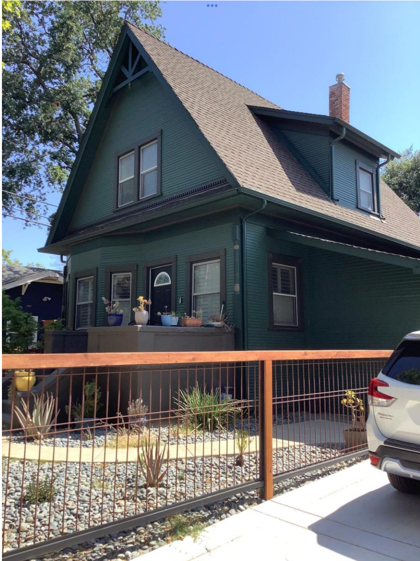
Photo 2: West facing street façade and south side of house with tool shed addition from 1964. The front door shown has been replaced with the original 1901 door.
