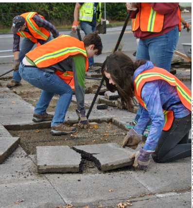
Depaving unused parking areas can lower surface temperatures and assist with stormwater management.
