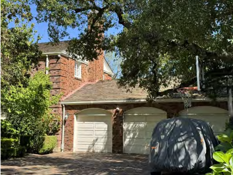
Photograph 3. View facing east, April 23, 2026.
