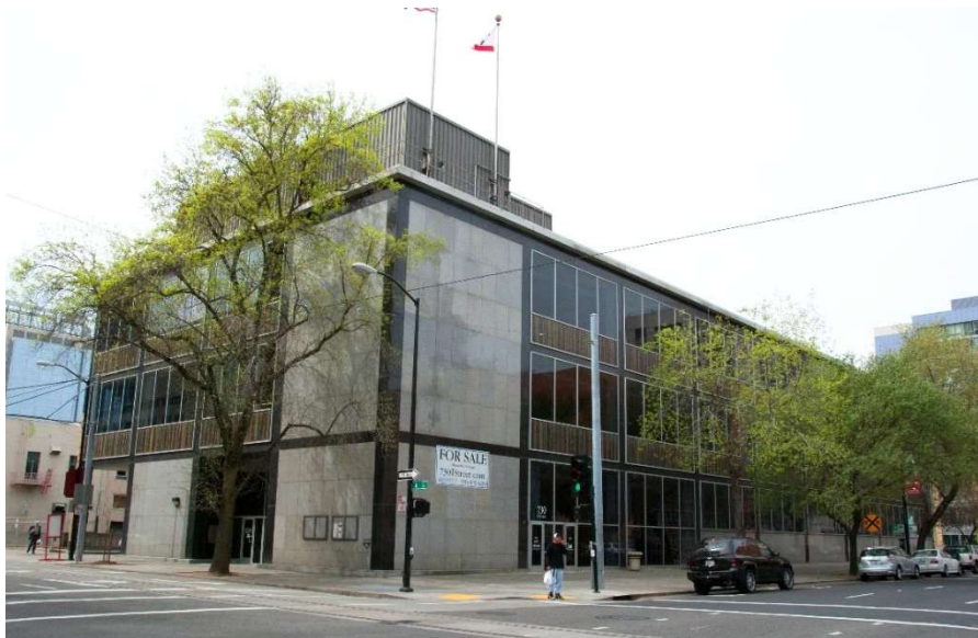
Figure 1: Bank of America Building at 730 I Street
