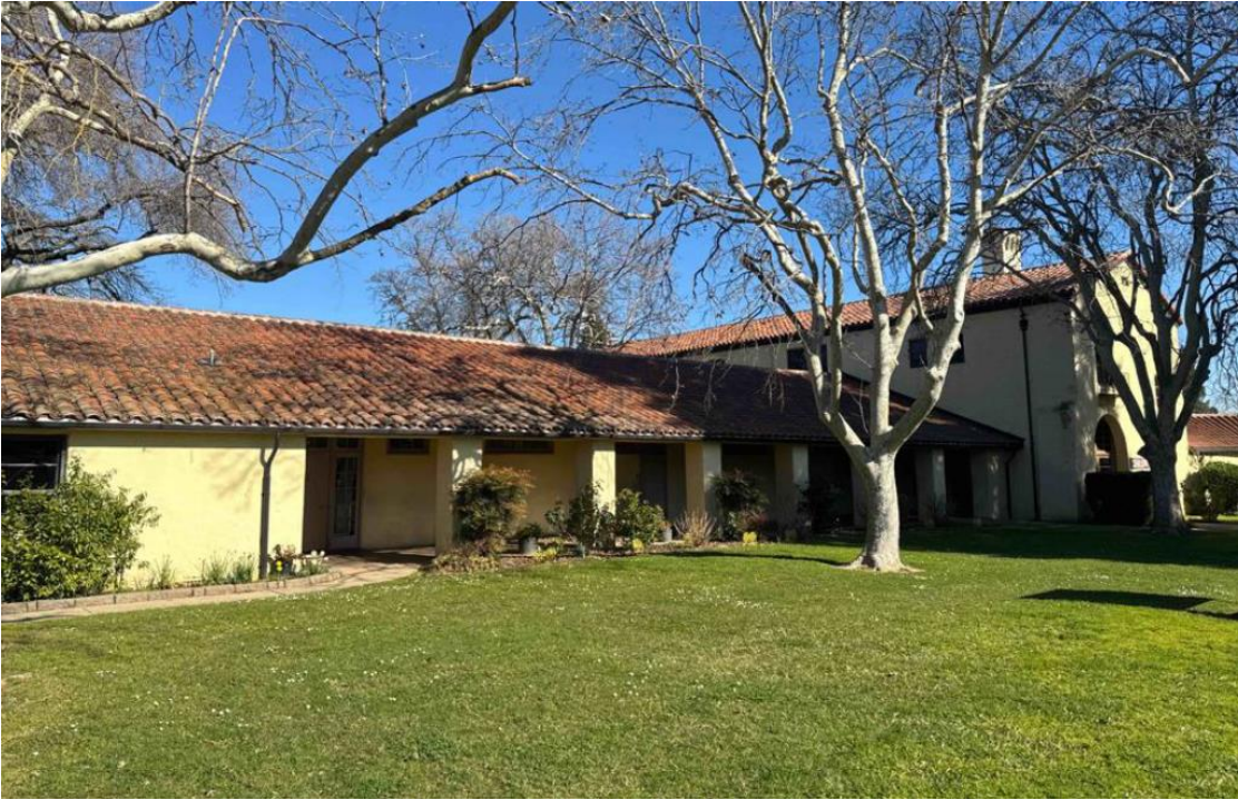
Figure 1: 5241 J Street, south and west elevations, view northeast
