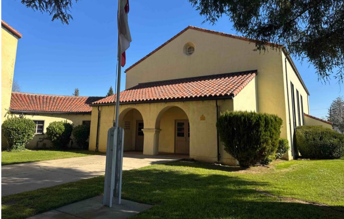
Figure 3: 5241 J Street, auditorium, view west
