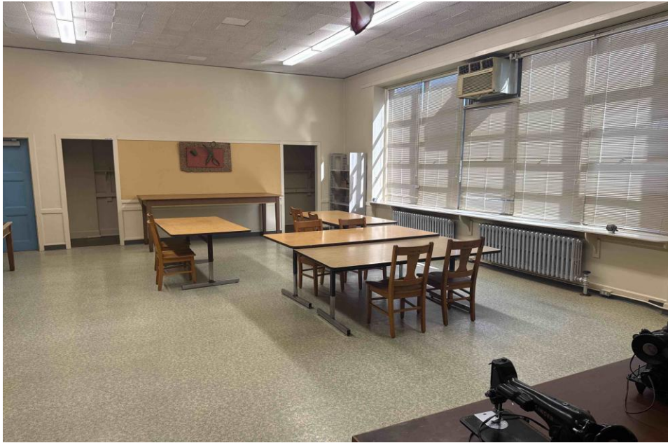
Photo 17 Classroom 10 (second floor) interior, camera facing northeast
