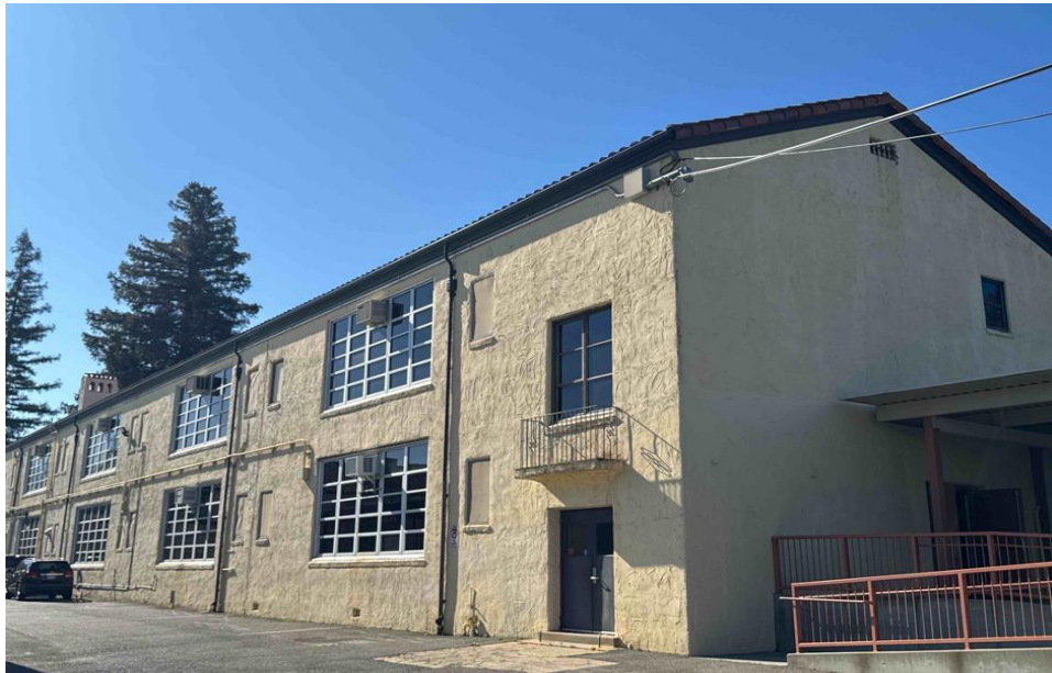
Figure 2: 5241 J Street, east and north elevations, view southwest
