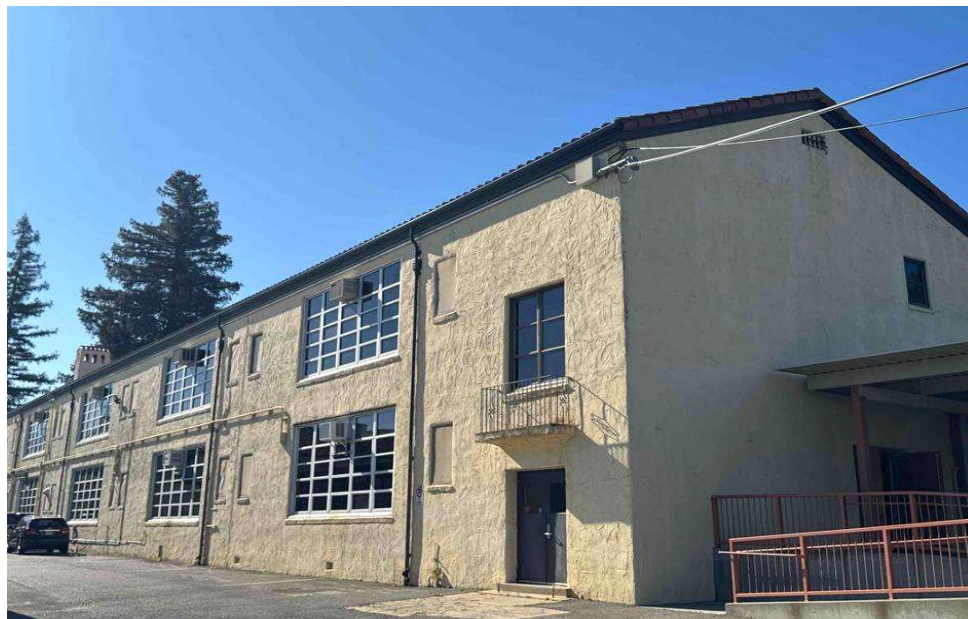
Figure 1: 5241 J Street (El Dorado School), south and west elevations, view northeast
