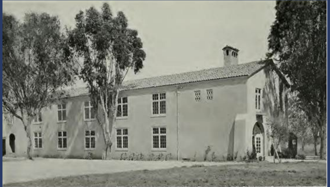
El Dorado School, 1922; Architect and Engineer, California
