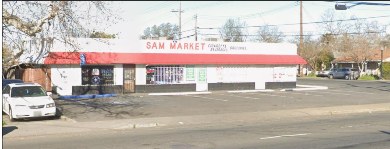
Figure 2: Existing Site Condition – Rio Linda Boulevard Street Frontage
