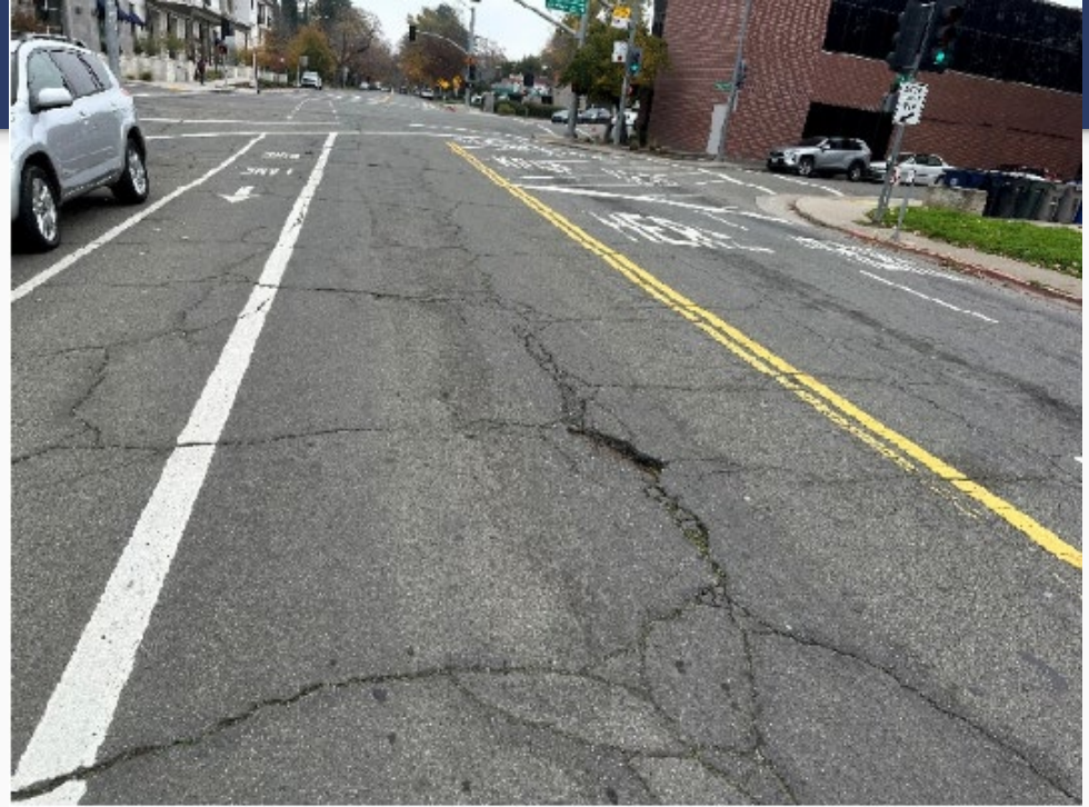
T Street: West of the Intersection with Gerber Ave
